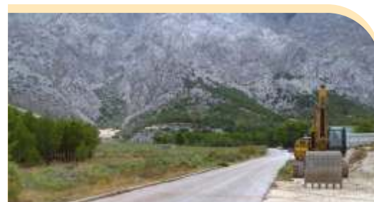
Construction of the link road
