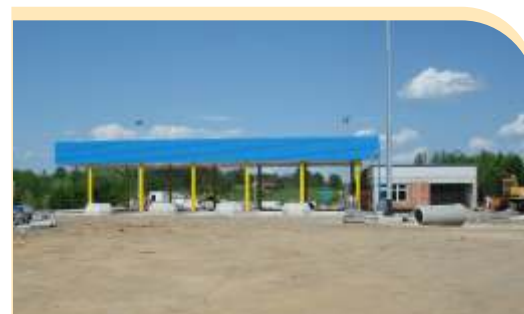
Novigrad Interchange in construction
